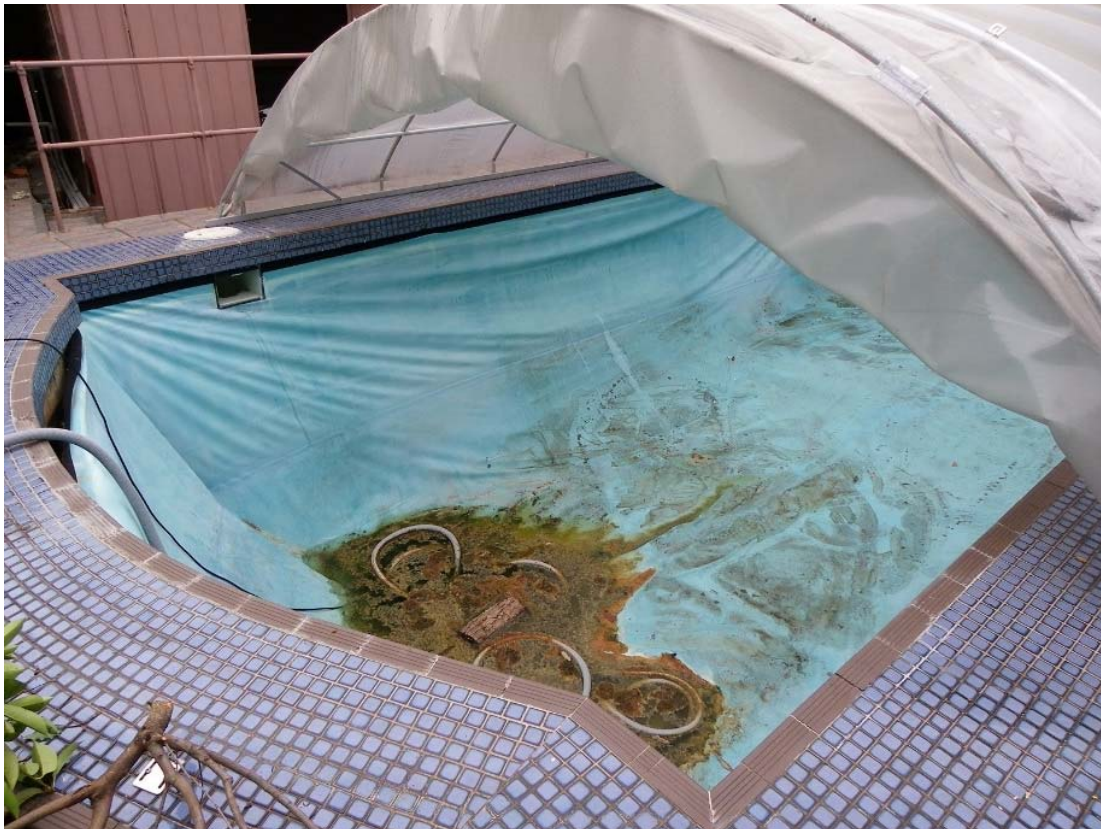
Pic 1. Here the liner has broken away from the fastenings and torn. Also, water has now got behind the liner making it difficult to use and providing an unhealthy water situation.
