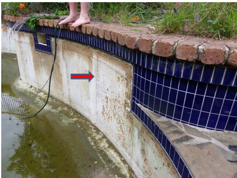
Pic 2 Depending on the shell construction upgrading with a coating (PaintnForget) is a better and much less expensive way to get the pool back into service. However if the shell is of panel construction then usually only an expensive liner can be reinstalled. Here we can see the panel joints (vertical lines) every metre along the wall, (arrow) meaning it probably can only have a new liner installed.
