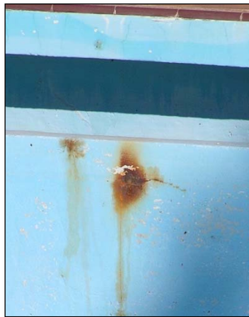
Crack with rust stains.
