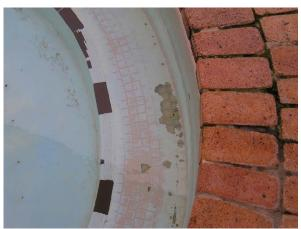
Fig2: (right) Painting of tiles is not recommended as it can lead to failure of the coating at the edges.
