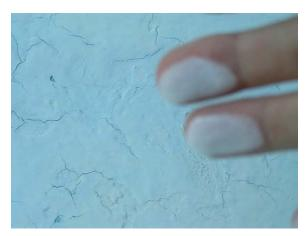
Fig 1: Paint can become chalky over time and leaves a film on your figures. This happens sooner with Chlorinated Rubber (1-2 yrs) and takes much longer with Epoxies. (5 -8 yrs) and for a MUCH longer life, (PaintnForget), which does not chalk. It may also be quite often the result of insoluble residues in your pool. Need to check which.
