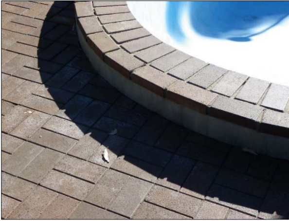
Figure 1 Dark pavers and coping with efflorescence present, with drainage. Resulted in blisters on pool walls
