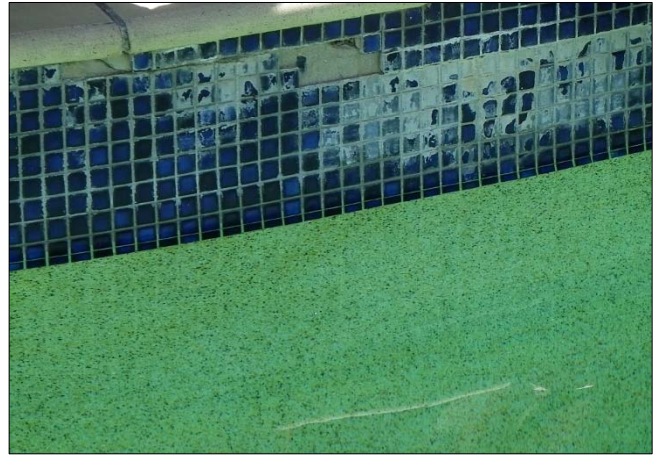
Figure 2 So many water related issues resulting in tiles being pushed off. Note area below tiles seems fine, as being porous.
