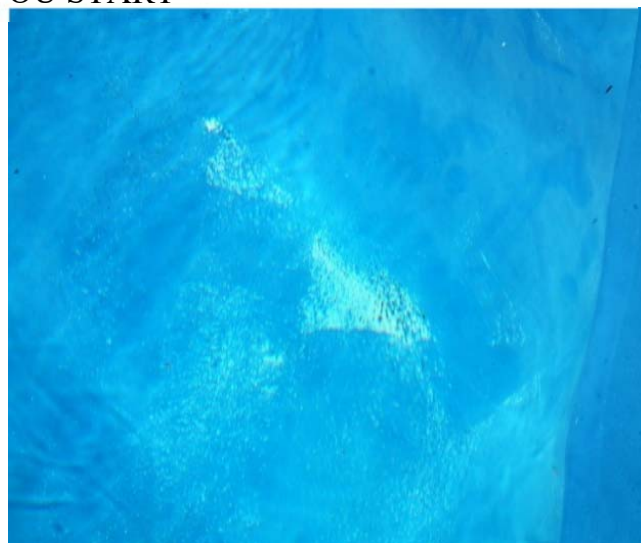
Figure 2. Not enough uniform spreading out, so worn off too soon in some areas.
