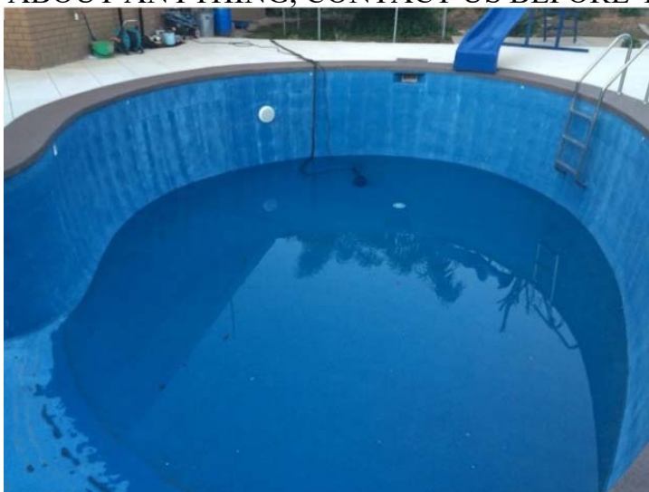
Figure 1. Vertical banding as no L to R spreading, only vertical.
