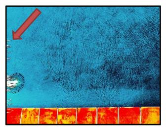
Here we can see "stains" moving away from the creepy crawler towards the right-hand corner where the surface is quite rough. The original pool surface area around the creepy crawler is quite smooth and thus clean as the coating is smooth also and follows the profile.
