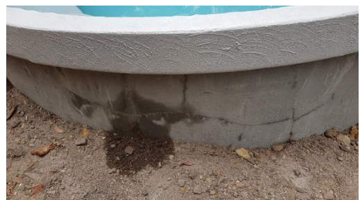
Fig 3: Leakage around skimmer box, probably due relative movement between pool and pipework as pool filled.
