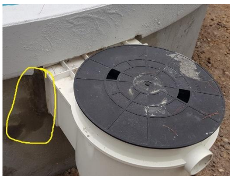
Fig 3: Leakage around skimmer box, probably due relative movement between pool and pipework as pool filled.
