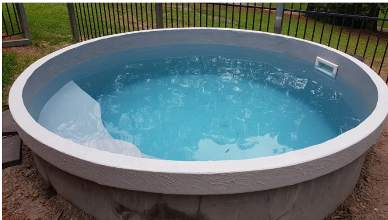
Fig 3: Leakage around skimmer box, probably due relative movement between pool and pipework as pool filled.
