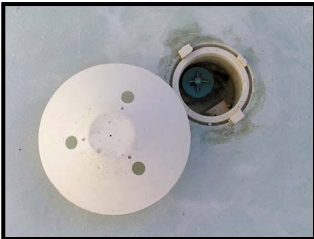
Fig 1: Typical hydrostatic valve assembly
